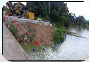
Installation of Silt Fence at the slope
