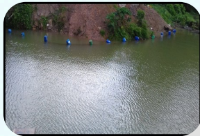
Installation of Silt Curtain at riverside
