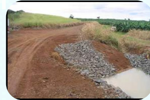
Implementation of Silt Trap
